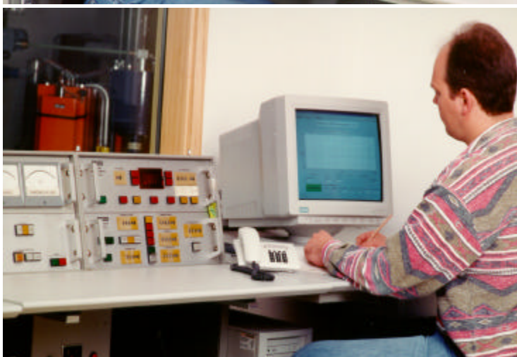
Fig.8b: Partial view to the control room at BET. The Personal Computer is underneath of the table. The Keyboard is protected by a metallic housing. A special screening of the PC and the Monitor is not required.
