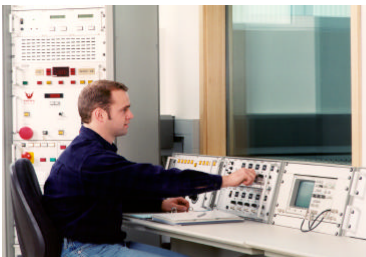
Fig.8a : Partial view to the control room at BET. The control unit for the HV Charging systems is on the left side inside the rack. The digital timing control unit is visible in the table. Next to it the commercial digital oscilloscope is installed.
